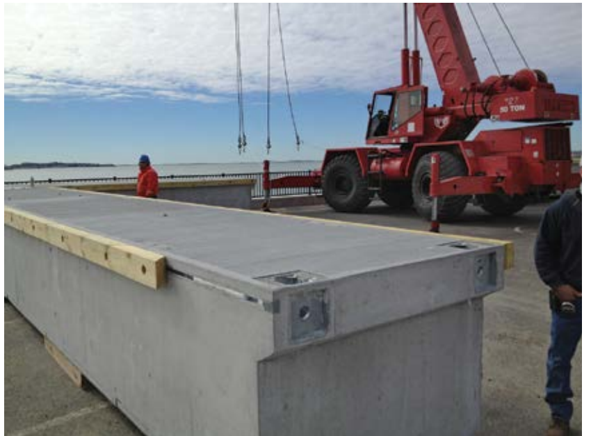
After arrival on site, many of the docks had to be floated by tugboats to their destinations, where they were lifted and lowered into place.
