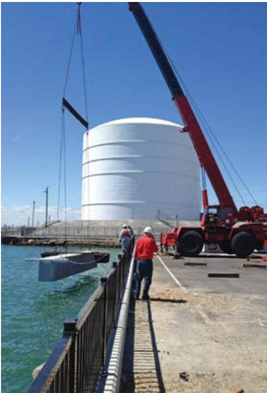
After arrival on site, many of the docks had to be floated by tugboats to their destinations, where they were lifted and lowered into place.
