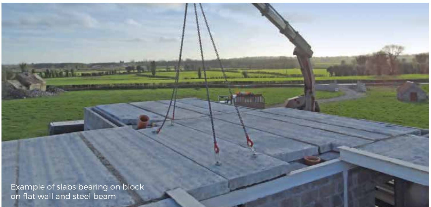
Slabs bearing on block wall
